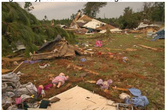
Fig. 46 Typical Tornado Damage
