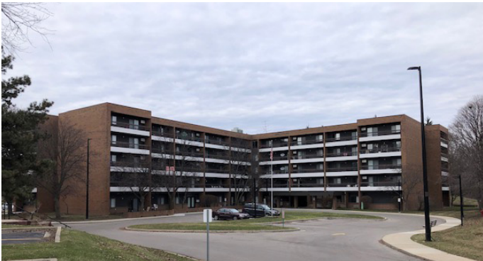
Senior apartment building.
