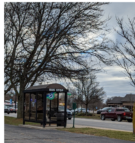
Bus stop on Aurelius Rd.
